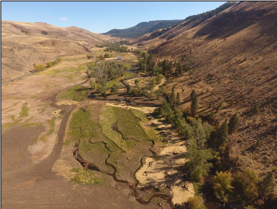
**FIGURE 10 CONSTRUCTION OF LARGE WOOD STRUCTURE AT LOWER PROJECT AREA.**
