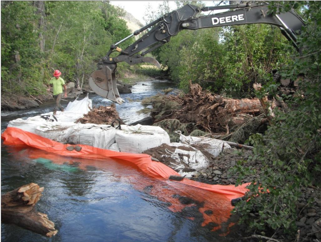
**FIGURE 11 CONSTRUCTION OF LARGE WOOD STRUCTURE AT UPPER PROJECT AREA.**
